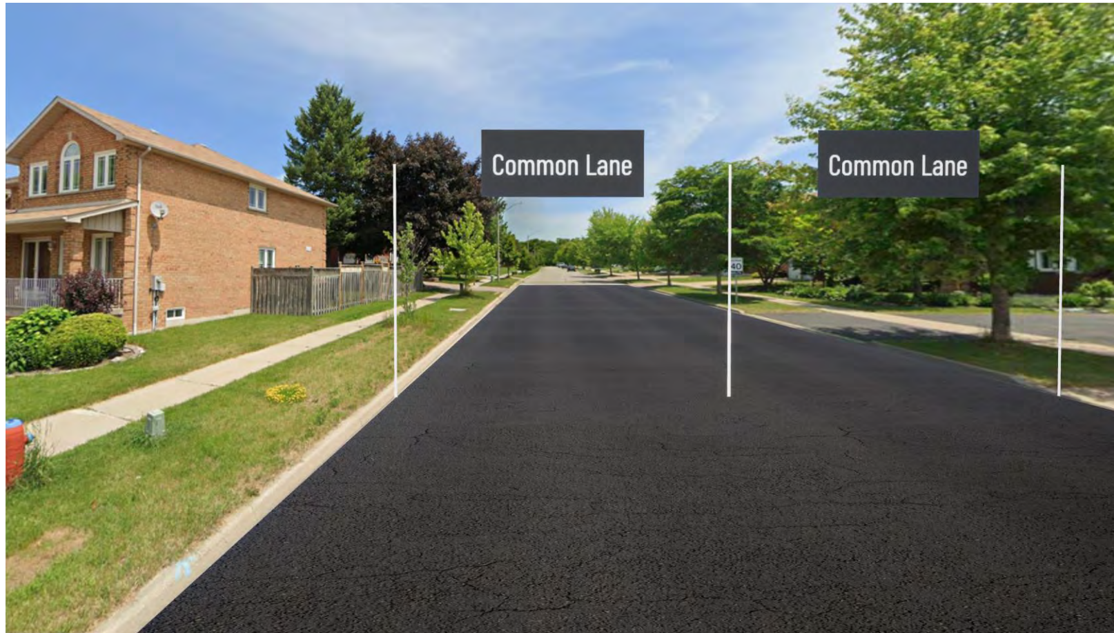
From Bayview Avenue To Edinburgh Drive – (Looking East)
