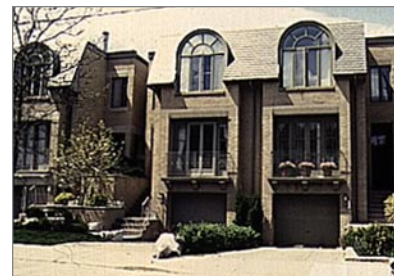
Driveway slightly sloped to reduce the elevation of the garage door, enabling the first floor to be closer to grade.
