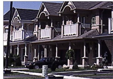
Port Union, porch overhangs extend across garage to reduce the visual dominance of garage doors.
