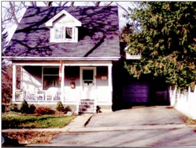
Dormer windows punctuate roof.
