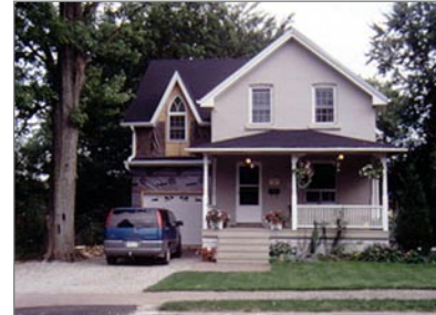
New garage located behind the front face of the building, with a second floor and roof that integrates with the primary building.
