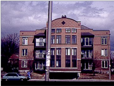
Buildings oriented to face the street. Access to underground parking is sloped to enable direct building to street relationship.
